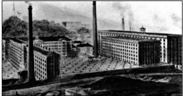
Above: The Dean Clough Mill Complex The Mill on the far right (Mill D) was the first designed by Ives
